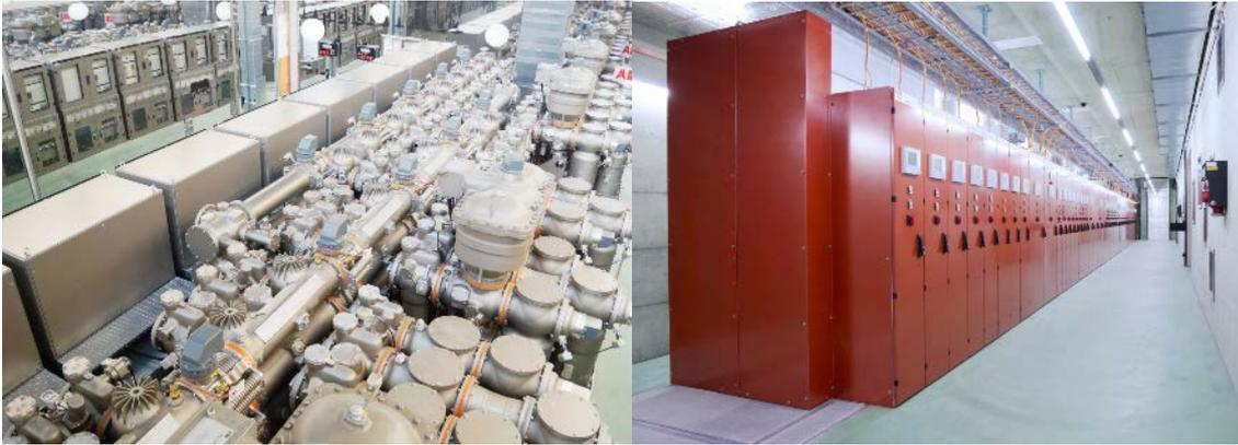
170 kV high-voltage GIS and 24 kV medium voltage GIS with eco-efficient gas mixture
