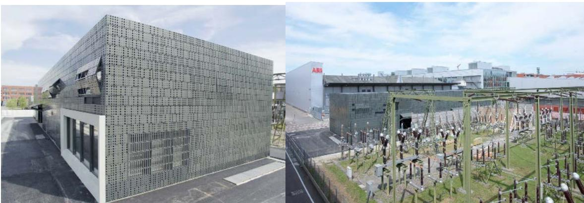
ewz substation in Oerlikon Zurich – the world's first pilot switchgear installation with eco-efficient gas mixture (right) replacing an aged air insulated switchyard with a 5x bigger footprint (left)
